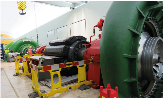
160 MW Happurg Pumped Storage Plant, Rehabilitation, Germany, 2020 – 2023
