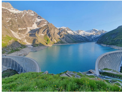
480 MW Limberg III Pumped Storage Plant (PSP), Austria, 2020 – 2024
