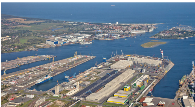
HyTech Hafen Rostock, Rostock, Germany, 2023 – 2024; 100 MW Electrolysis Plant at the existing coal-fired Power Plant in Rostock.
