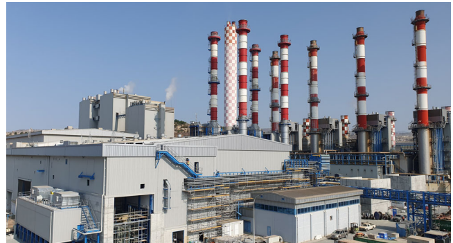
868 MW Vasilikos Combined Cycle Power Plant, Cyprus, 2019 – ongoing
