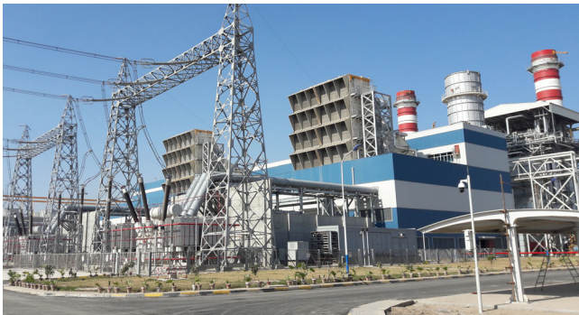
Three Combined Cycle Power Plants (CCPP) Balloki, Haveli Bahadur Shah and Bhikki, Pakistan, 2015 – 2018. One of the world's highest efficiencies of 63% is achieved in the Haveli Bahadur Shah CCPP with H-class gas turbines.
