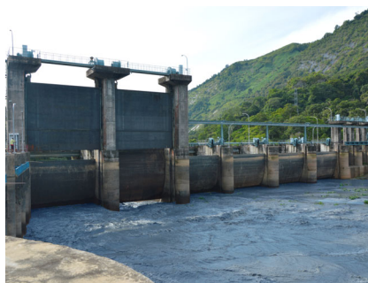
270 MW Bakaru I & II Hydropower Plant, Indonesia, 2020 – 2023
