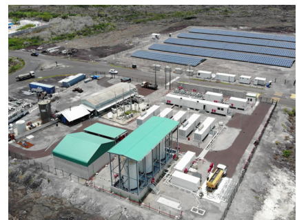
Hybrid Power Plant Jatropa / Diesel & PV & BESS, Galapagos, Ecuador, 2010 – 2021
